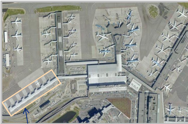
H/M pier Low Cost
