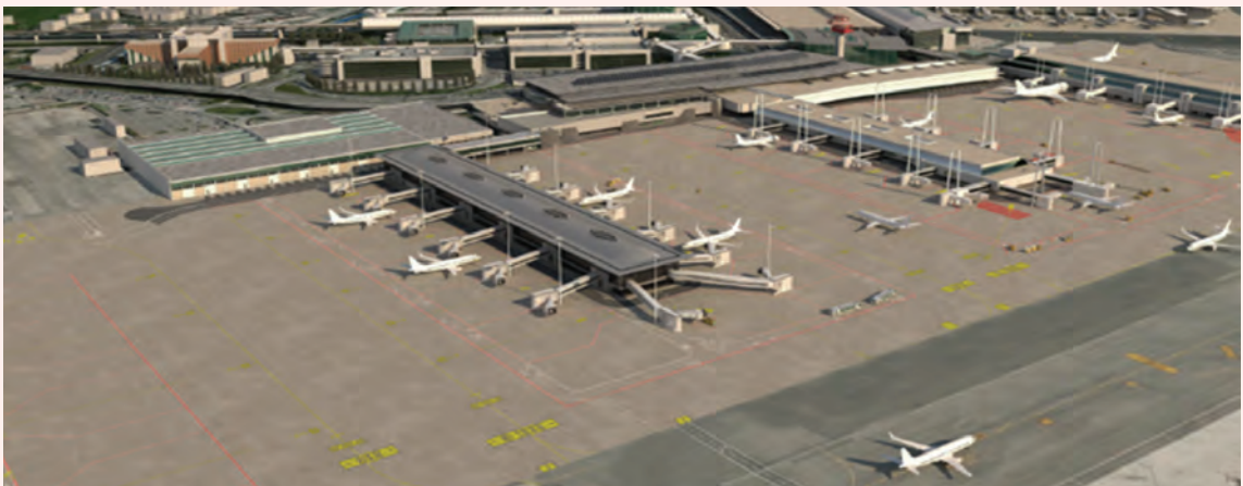
Terminal system area-east – Overview
