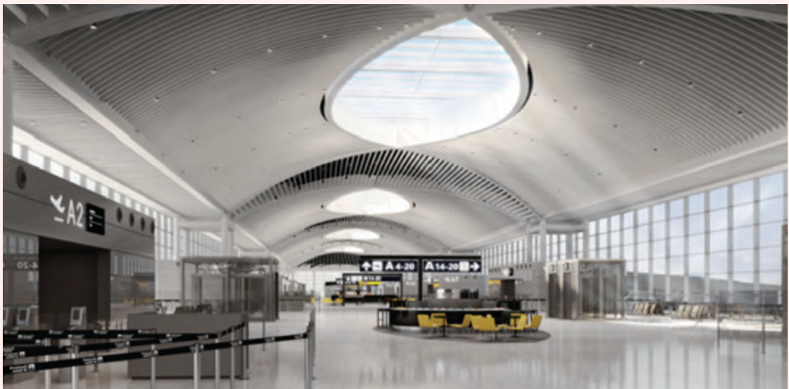
New Pier A
